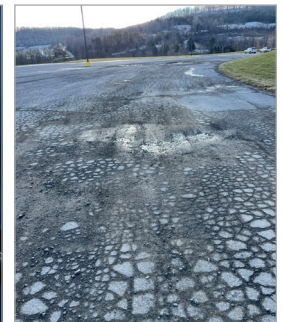
Reconstruct south parking lot
