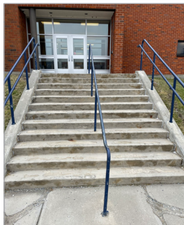
Replace elementary entrance stairwell
