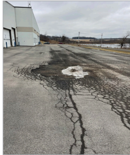
Reconstruct asphalt pavement
