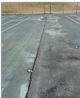
Resurface tennis courts
