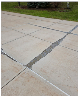
Reconstruct elementary/main entrance sidewalk
